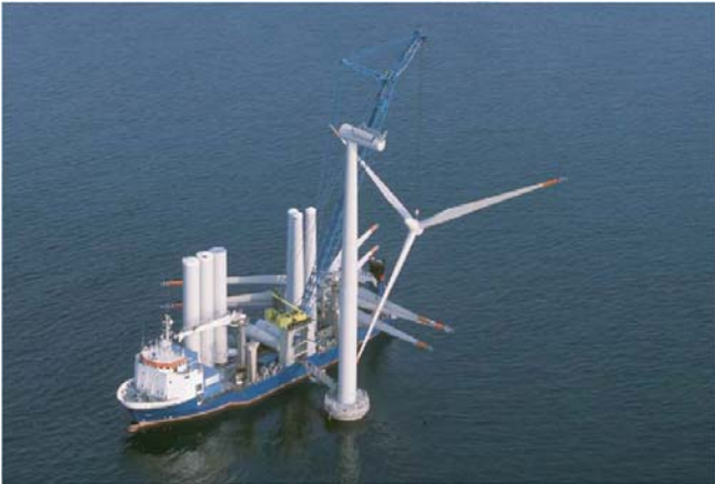
Installation vessel; source: A2Sea Management Report 2003
