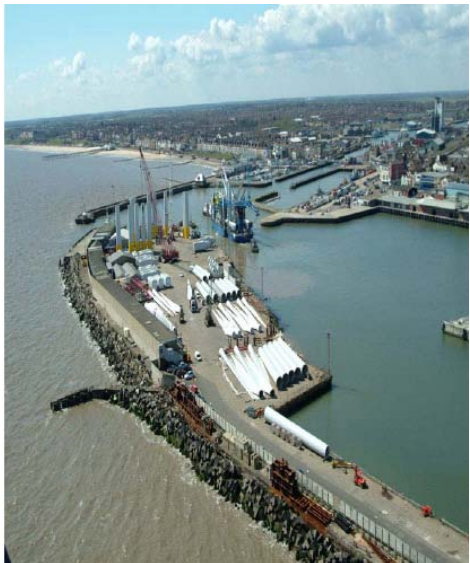
Elements at quayside; Source: E.ON UK, Chatterton
