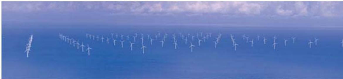
Figure 7-1: View of the Horns Rev wind farm.
