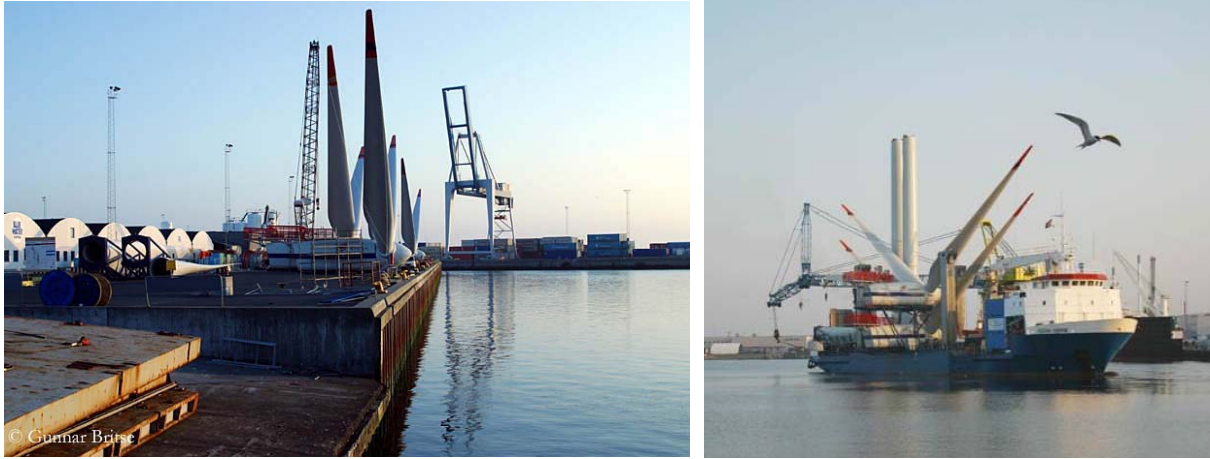
Figure 7-17: Turbine assembly area in the harbour and shipping out of the harbour (Source: Gunnar Britse).
