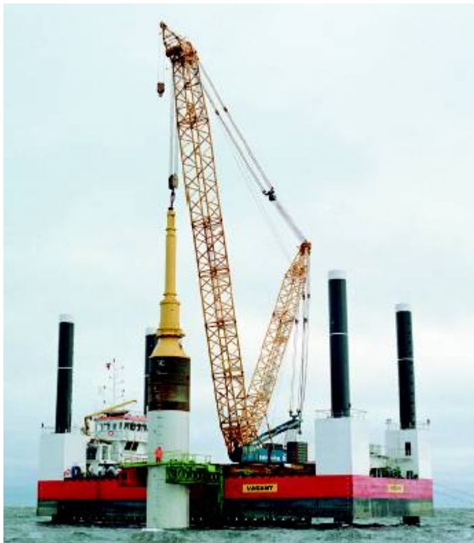
Figure 3-4: Vagant Jack-up platform used for soil investigations.
