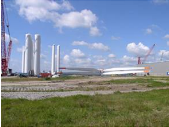
Area for pre assembly; Source: dena
