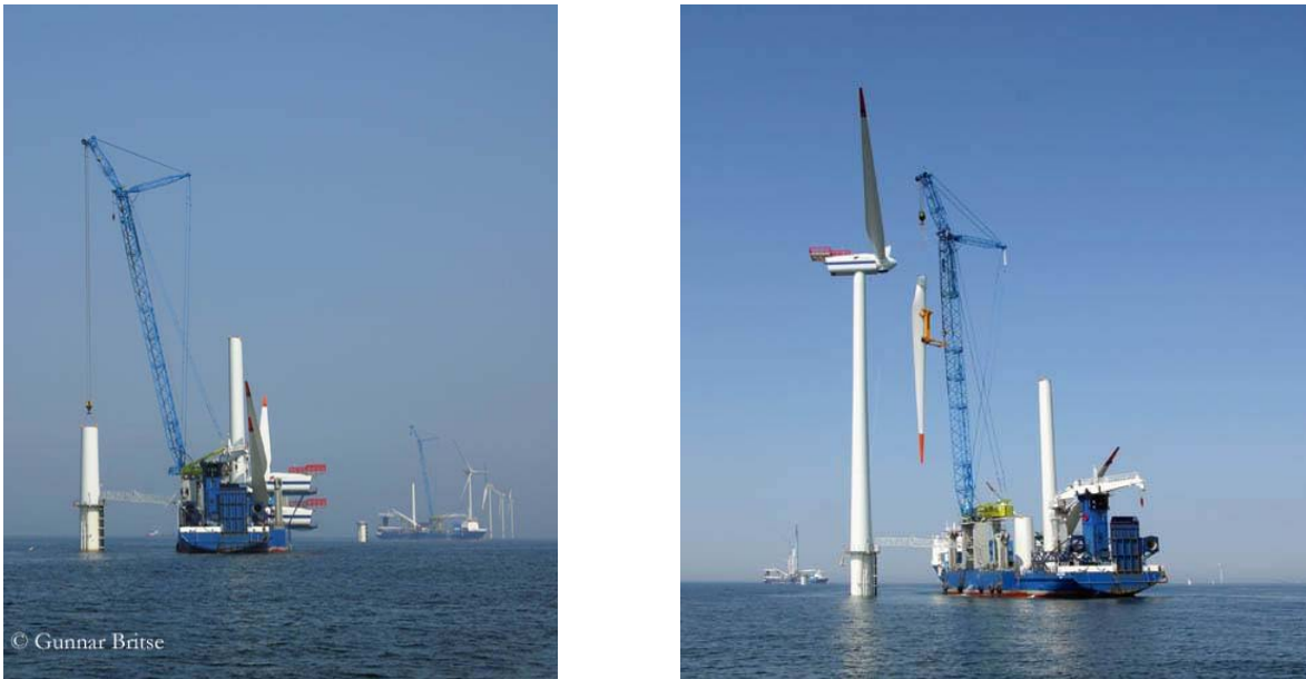
Figure 7-18: Installation of tower (left) and rotor blades (right) (Source: Gunnar Britse).
