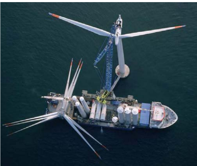
Installation vessel A2Sea; Source: Siemens Wind Power 70
