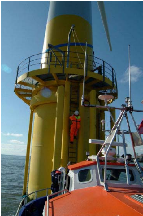
Access to pile; source: E.ON-UK 131
