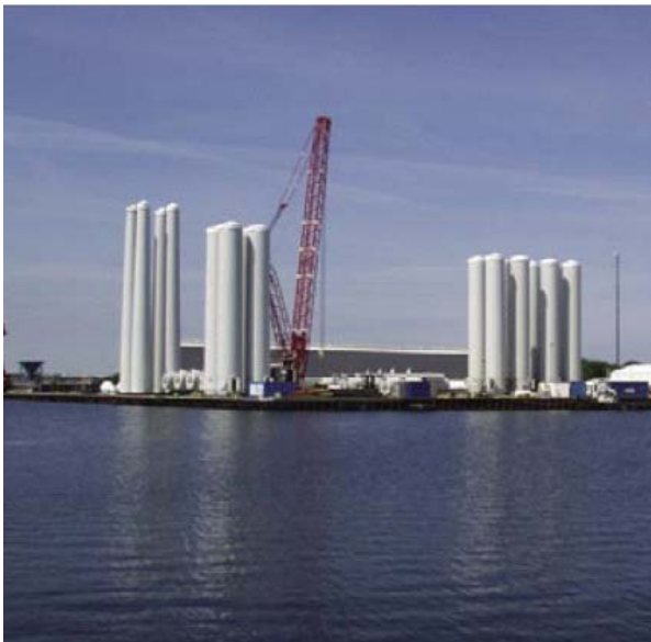
Material at quayside; Source: Offshore Centre Denmark 78
